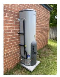
Storage water units are just that – they store hot water for use when your home needs it. Gas Storage hot water units use a gas burner to continuously heat and maintain water at approximately 60 °C. Sufficient ventilation is also required for these systems.
