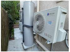
A Heat Pump system has some similarities to an Electric Storage system, they both have a tank and use electricity as the source for the heat. However, instead of an element to heat the water, a heat pump extracts heat from the ambient air to heat to the water. They can operate in temperatures as low as minus 10 degrees Celsius. The main advantage of this system compared to the Electric Storage system is that it uses significantly less electricity. These systems can
