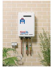
As the name suggests these systems heat water as you need it. The system works by having cold water flow through copper piping, and heat is then applied directly to the pipes. A continuous flow of gas and sufficient ventilation is required for this system.
