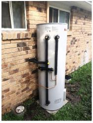
Storage Electric hot water systems are one of the most commonly used systems in Australia, including in the majority of apartment and unit blocks. They work similar to a Gas Storage system except they use electricity and an element to heat the water.
